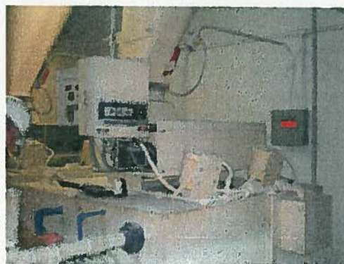
Figure 4-23: Fluoride Feeders
