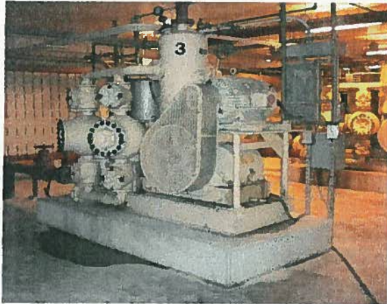
Figure 4-29: High Pressure Pump
