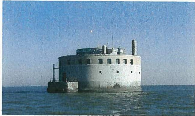
Figure 4-9: Raw Water Intake
