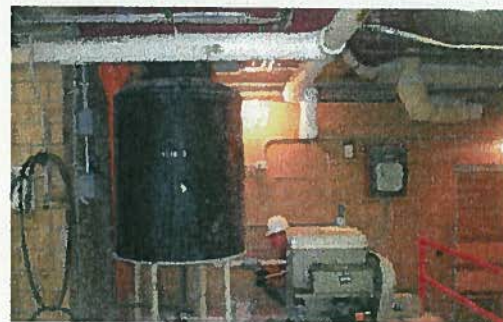
Figure 4-19: Alum Day Tank and Rotadip Feed System
