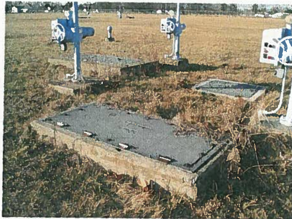
Figure 4-33: Concrete On Top of Reservoirs
