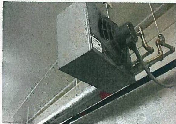
Figure 4-45: Exhaust Fan in Residuals Handling and Dewatering Facility
