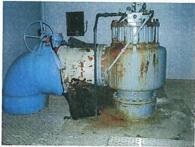
Figure 4-30: Waste Washwater Pump
