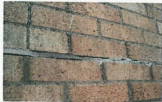
Figure 4-37: Cracking in Brick Structures
