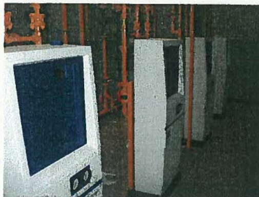
Figure 4-22: Chlorinators
