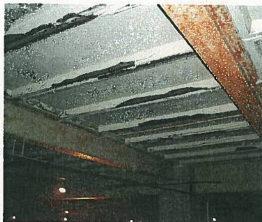
Figure 4-32: Concrete Roof Deck In Flocculation/Sedimentation Area
